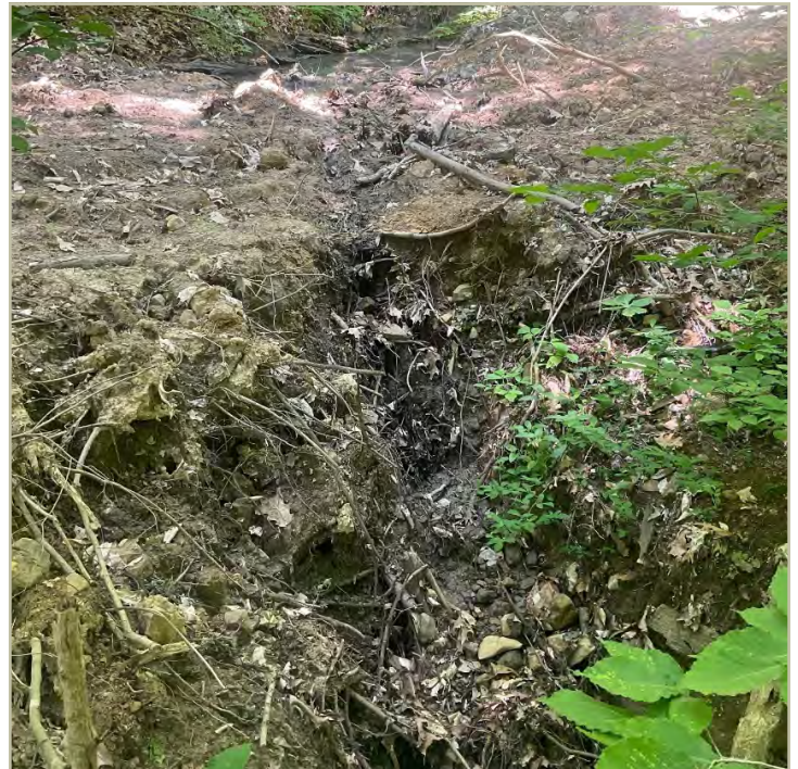
Soil was pushed into this ephemeral stream to allow a skid trail to cross. The soil was not removed after harvest completion and now the ephemeral is backing up and running over the trail during precipitation events, causing sediment to enter the watershed.
