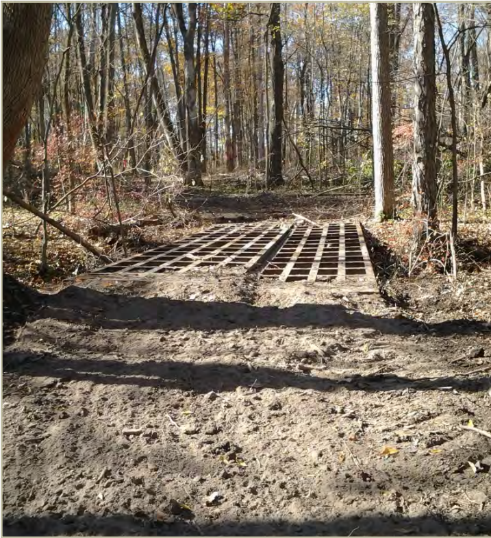
This metal grate bridge protects stream banks.
