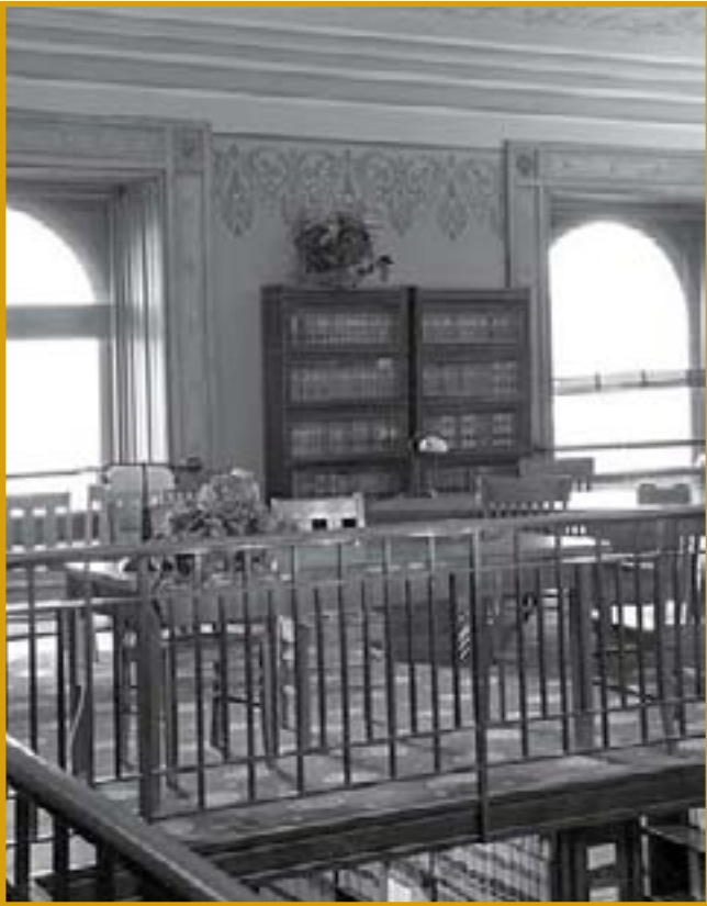
★ The mezzanine level in the renovated Library.
