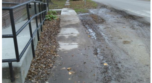
Before construction began
