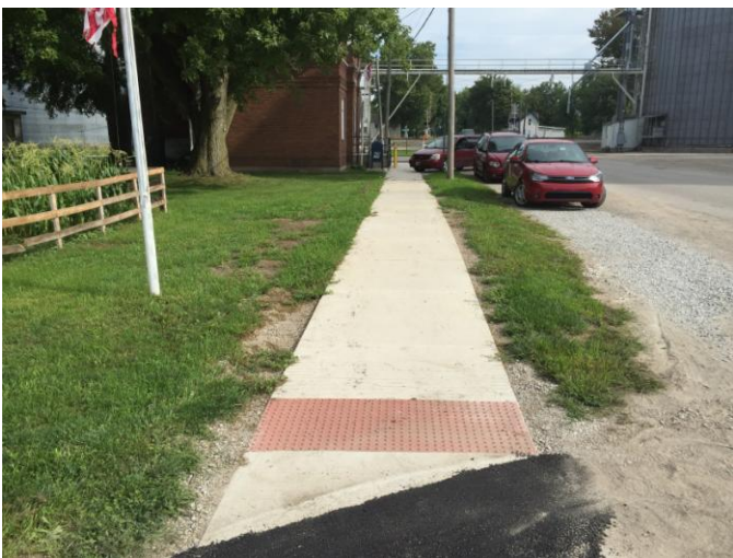
Asphalt was placed to match the concrete to the road.
