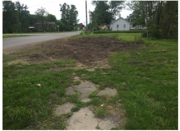
After Tree removal and stump grinding
