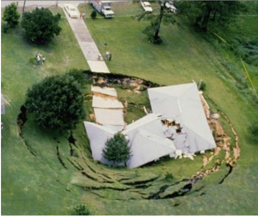
Figure 3-20 Home Swallowed by Land Subsidence
