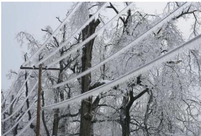
Figure 3-23 Ice Covered Power Lines
