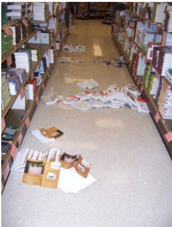
Figure 3-7 Minor Earthquake Damages
