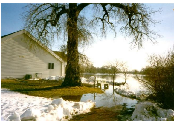
Figure 3-26 Flooding Caused by Snow Melt
