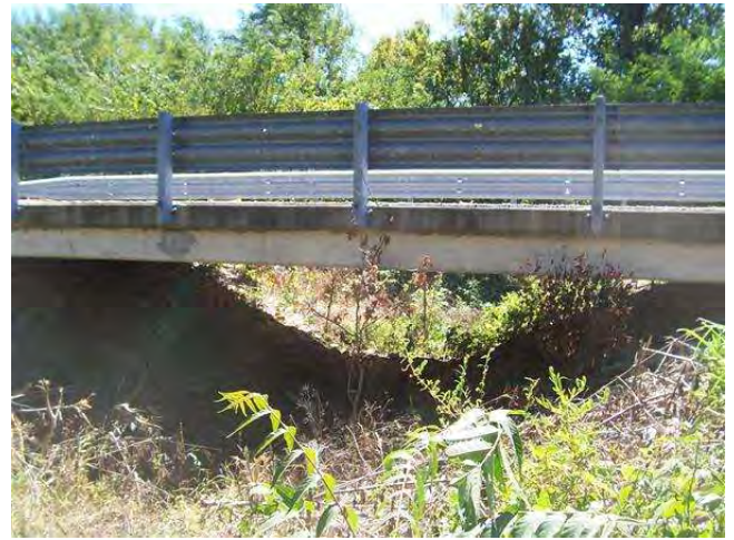
LOOKING SOUTH IN CHANNEL
