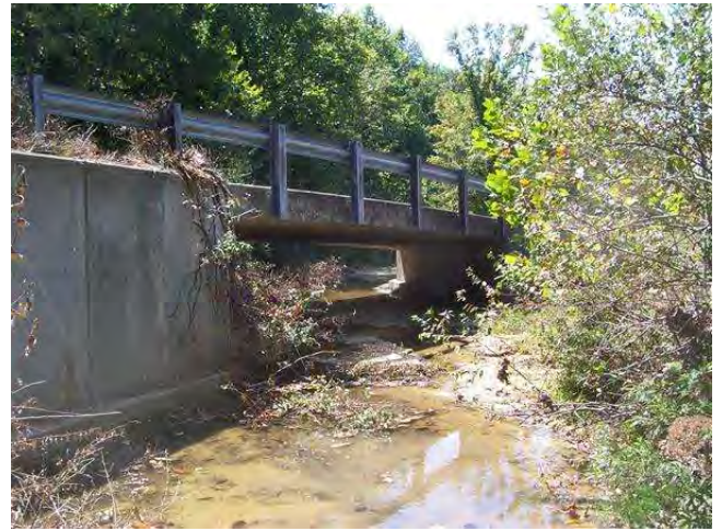
LOOKING SOUTH IN CHANNEL
