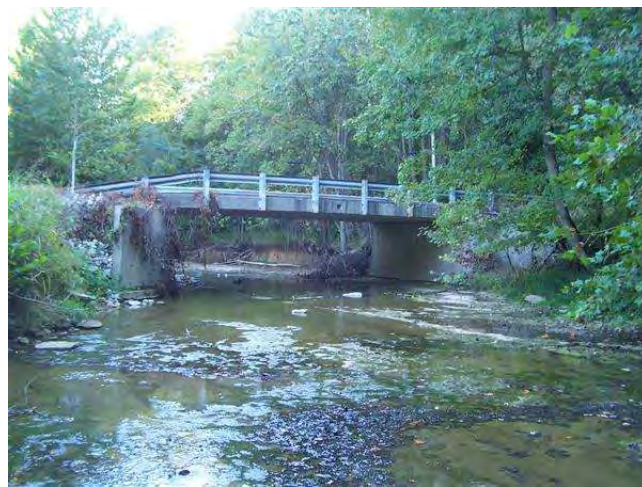
LOOKING SOUTH IN CHANNEL
