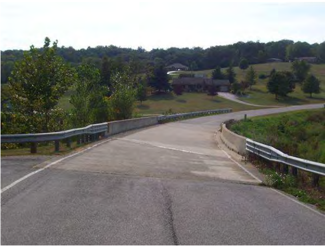
LOOKING WEST ON ROAD
