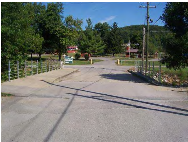
LOOKING NORTH FROM ROAD
