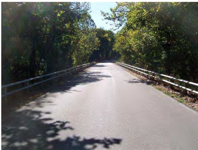
LOOKING WEST ON ROAD
