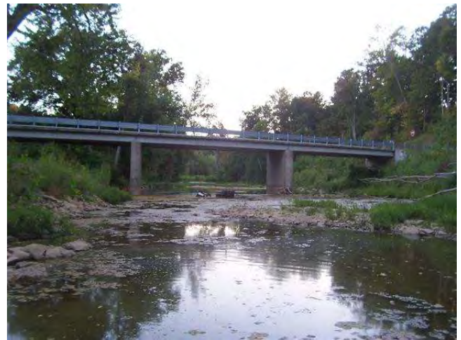
LOOKING SOUTH IN CHANNEL
