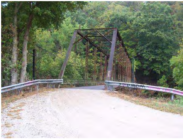
LOOKING WEST ON ROAD
