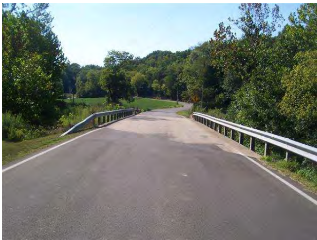
LOOKING WEST ON ROAD
