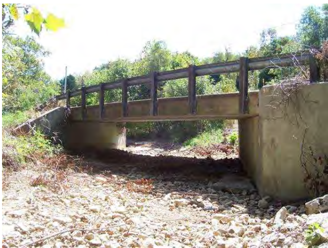
LOOKING SOUTH IN CHANNEL
