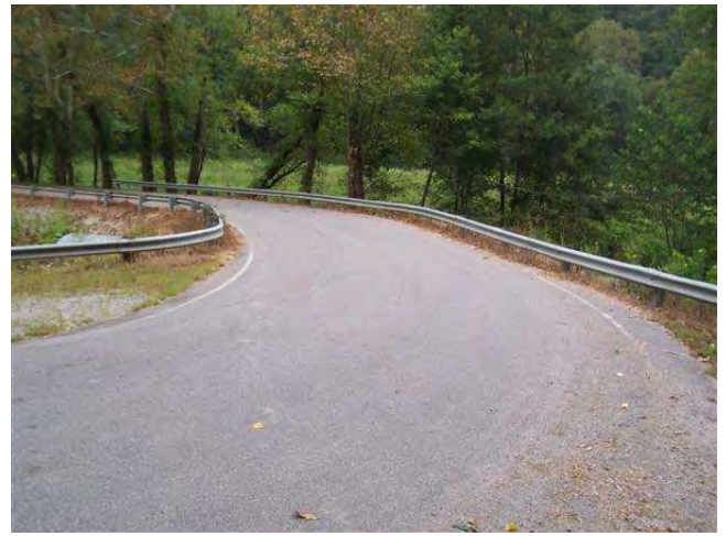
LOOKING WEST ON ROAD
