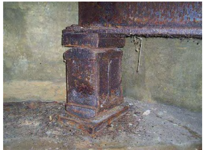
BEAM #5 BEARING AT BENT #4
