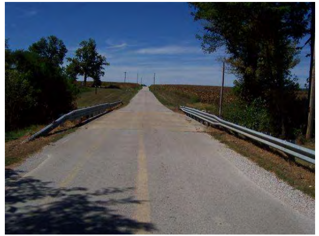
LOOKING WEST ON ROAD
