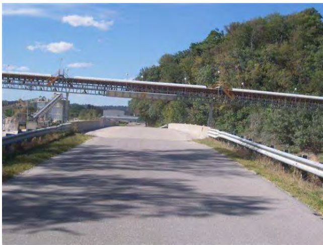
LOOKING WEST ON ROAD
