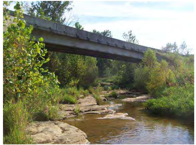
LOOKING SOUTH IN CHANNEL
