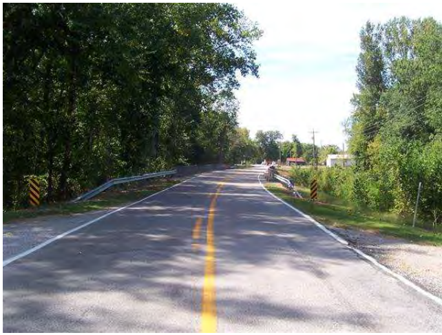
LOOKING WEST ON ROAD
