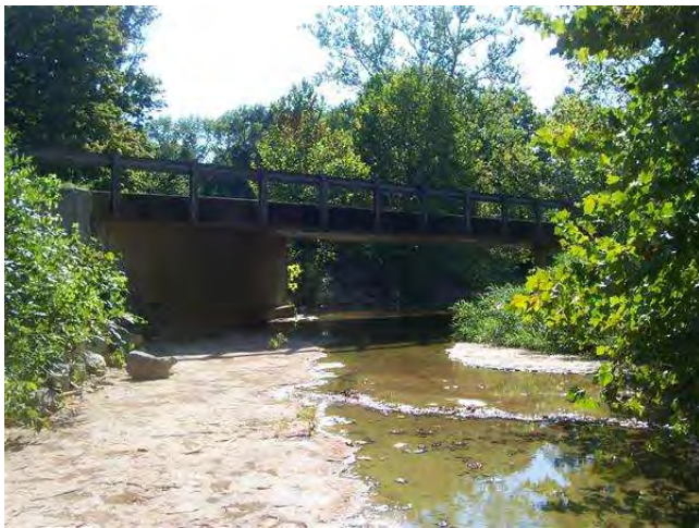
LOOKING SOUTH IN CHANNEL
