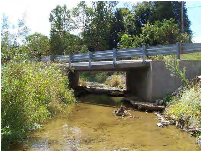
LOOKING SOUTH IN CHANNEL
