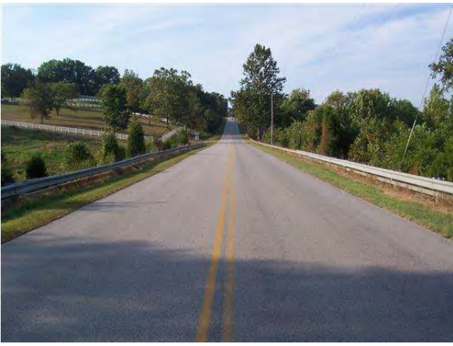
LOOKING NORTH ON ROAD
