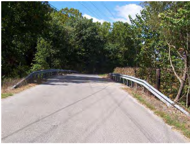
LOOKING WEST ON ROAD
