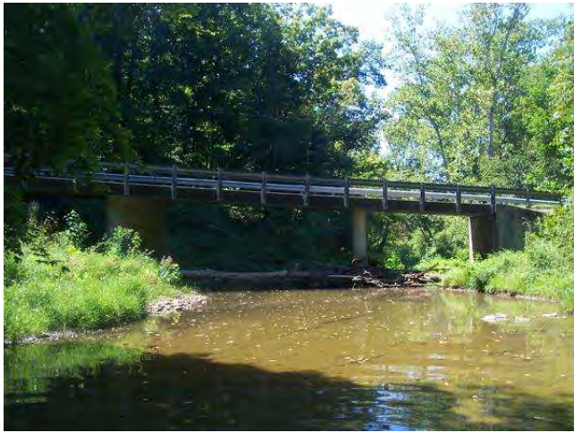
LOOKING SOUTH IN CHANNEL
