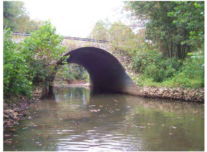
LOOKING SOUTH IN CHANNEL
