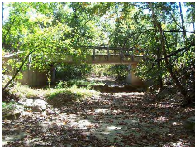
LOOKING SOUTH IN CHANNEL
