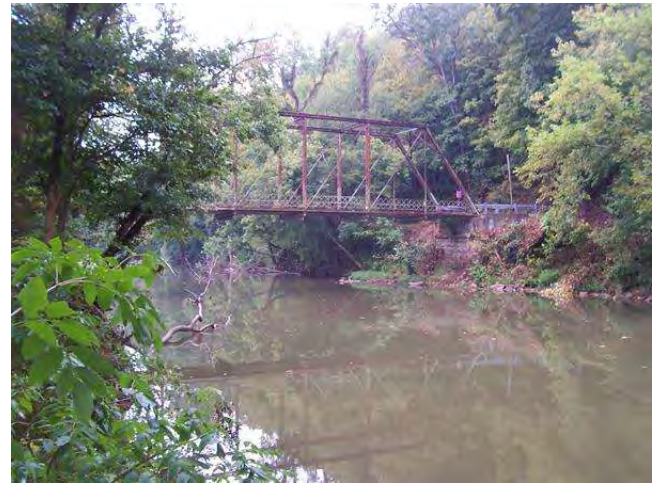
LOOKING SOUTH IN CHANNEL
