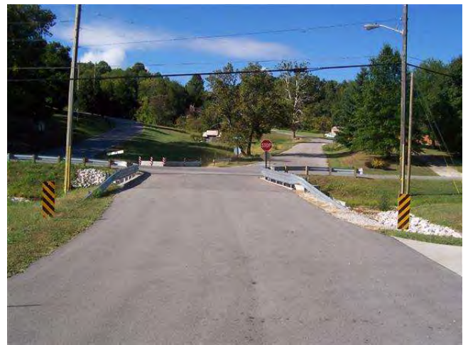
LOOKING WEST ON ROAD
