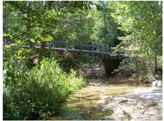
LOOKING SOUTH IN CHANNEL
