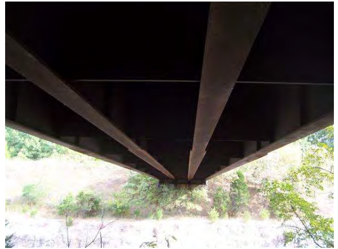
LOOKING NORTH AT BOTTOM OF SUPERSTRUCTURE
