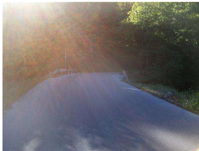
LOOKING WEST ON ROAD
