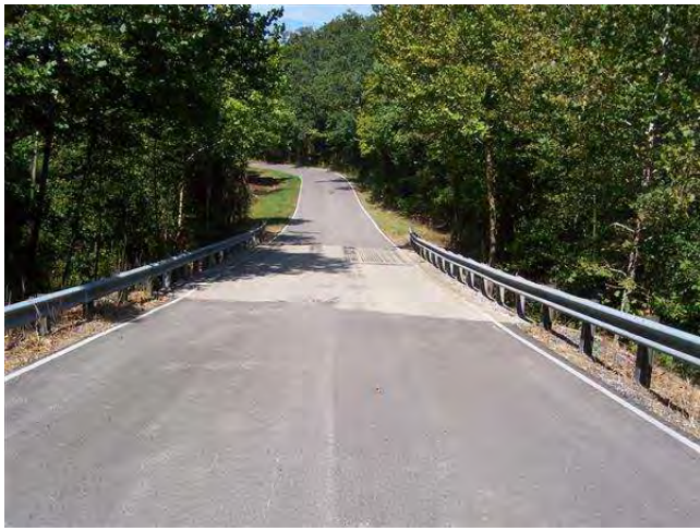
LOOKING WEST ON ROAD
