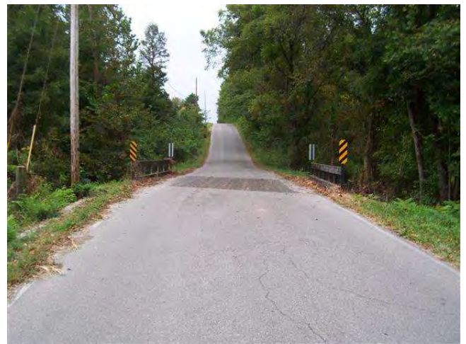
LOOKING SOUTH ON ROAD
