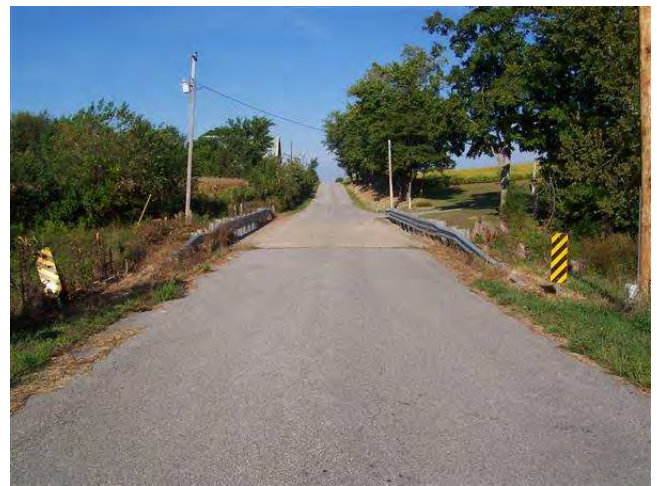
LOOKING WEST ON ROAD
