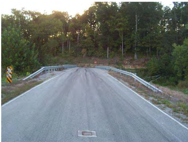
LOOKING WEST ON ROAD
