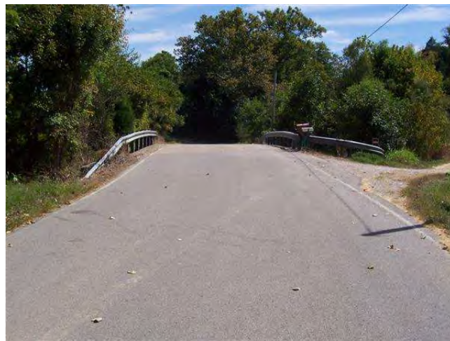
LOOKING WEST ON ROAD
