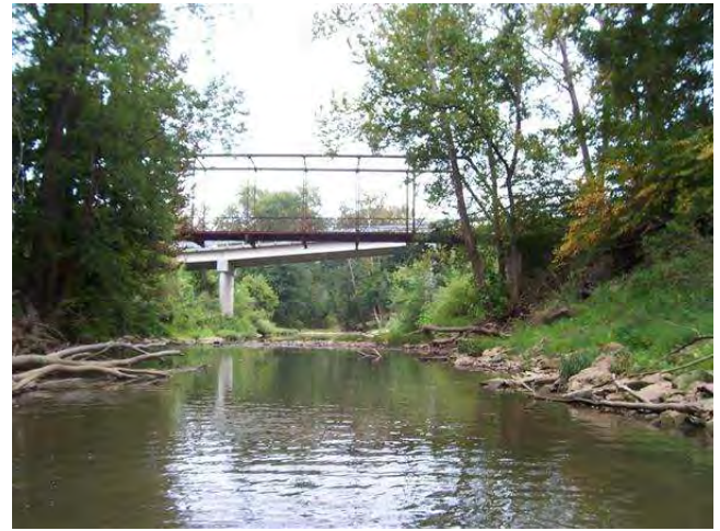
LOOKING SOUTHEAST IN CHANNEL
