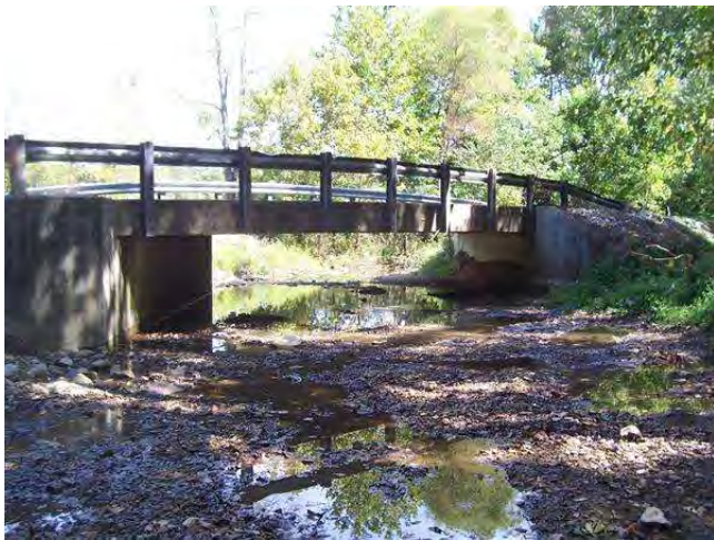
LOOKING SOUTH IN CHANNEL
