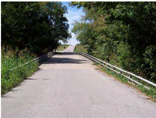
LOOKING WEST ON ROAD
