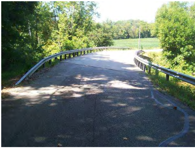
LOOKING WEST ON ROAD
