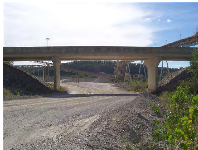
LOOKING SOUTH FROM ROAD
