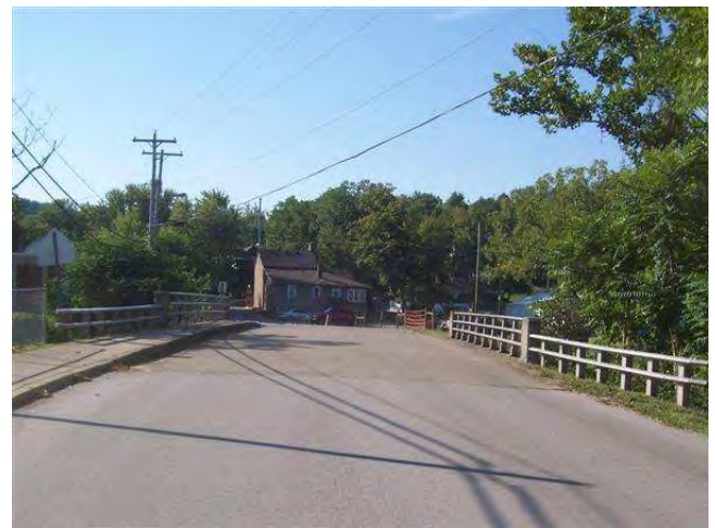
LOOKING SOUTH FROM ROAD
