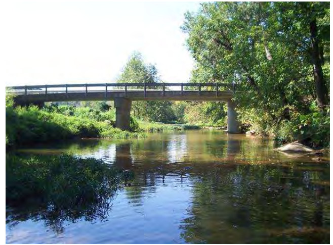
LOOKING SOUTH IN CHANNEL
