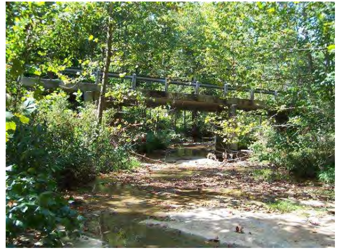
LOOKING SOUTH IN CHANNEL
