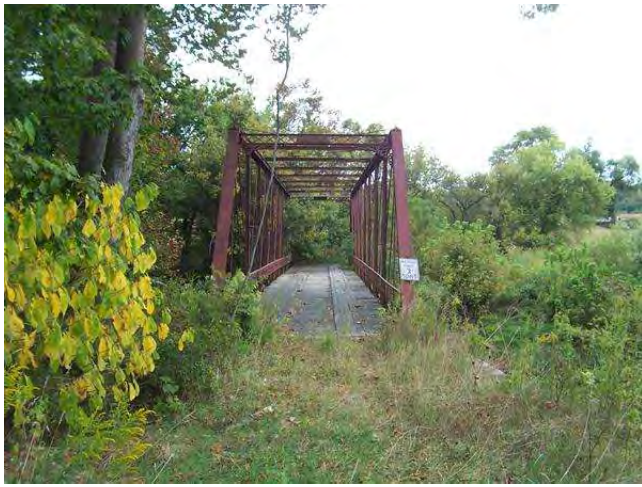
LOOKING NORTHEAST ON ROAD
