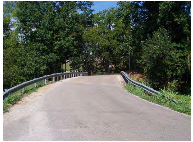
LOOKING WEST ON ROAD
