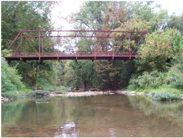
LOOKING NORTHWEST IN CHANNEL
