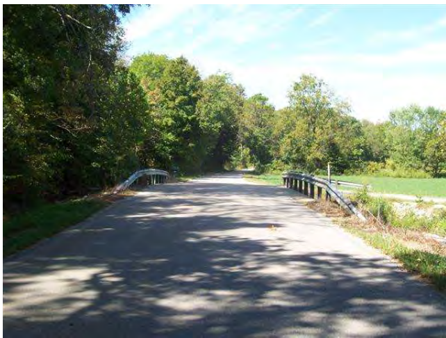
LOOKING WEST ON ROAD
