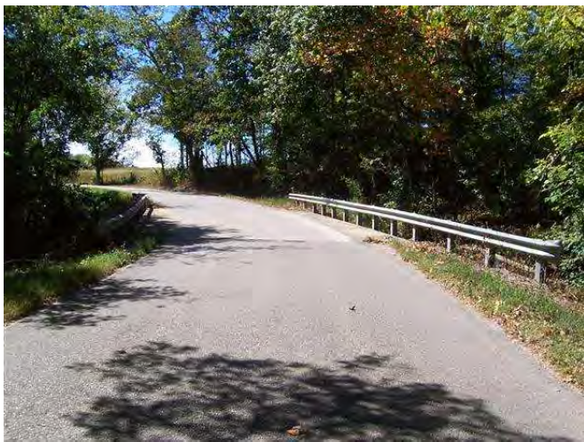
LOOKING WEST ON ROAD
