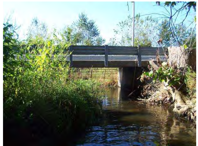
LOOKING SOUTH IN CHANNEL
