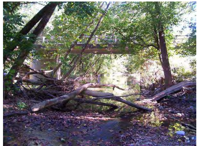
LOOKING SOUTH IN CHANNEL
