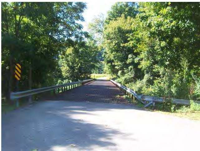
LOOKING SOUTH FROM ROAD
