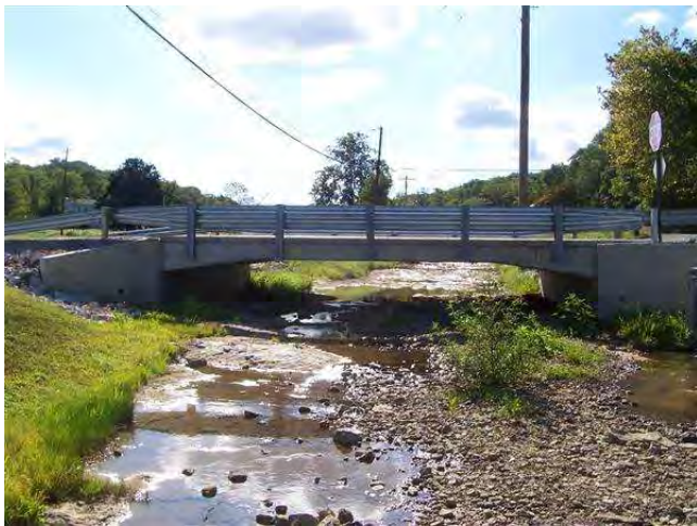
LOOKING SOUTH IN CHANNEL
