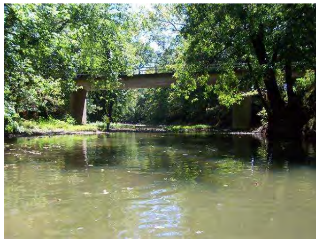
LOOKING SOUTH IN CHANNEL
