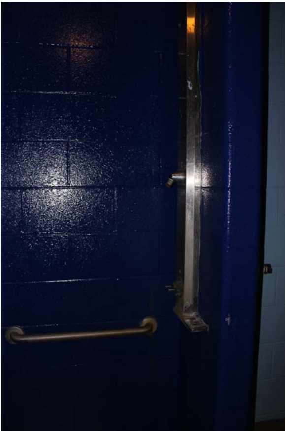
The shower head and controls while mounted on the correct wall are too close to the adjacent wall. The grab bars are in a non-compliant configuration.
